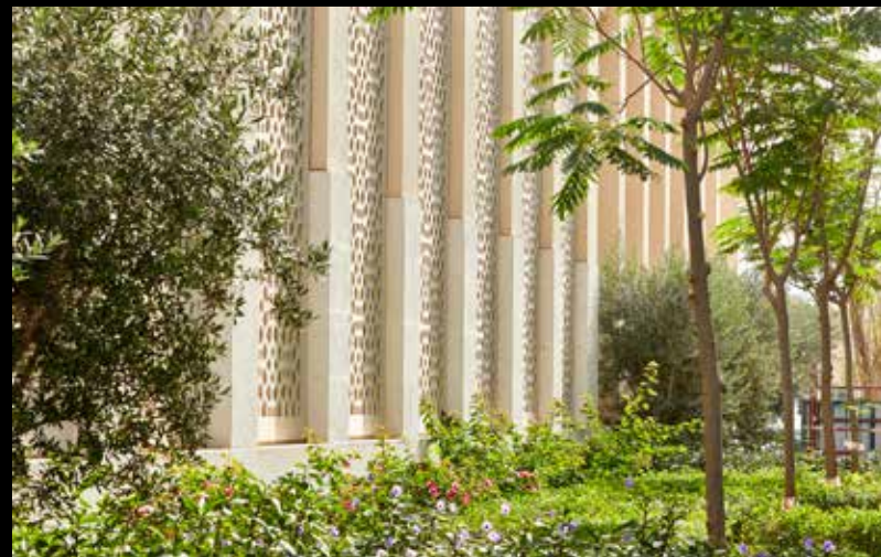
above: Religious life is an important part of the city dynamic, so the district includes three mosques where residents pray several times a day. These sacred structures are by John McAslan + Partners (left and top right) and Allies and Morrison (bottom right).
